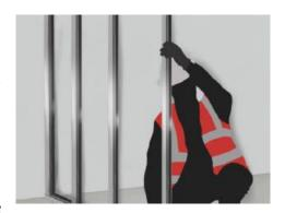
For heights that exceed the maximum manufacturer stud length, the Hadley I Studs would require to be spliced as per our recommended splicing detail. DRY-HAD-XX-ZZ-DT-X-1912
