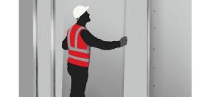
Plasterboard should be Screw fixed at maximum 300mm centres with centres reduced to 200mm at all corners.
